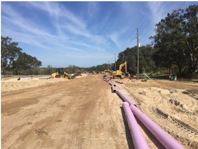
New infrastructure being constructed along Hull Island Road.
