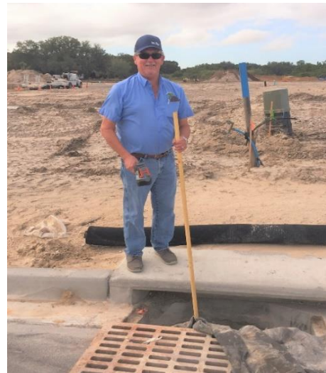
Public Works employee, Wayne Tallman, inspecting drainage facilities at Oakland Park.
